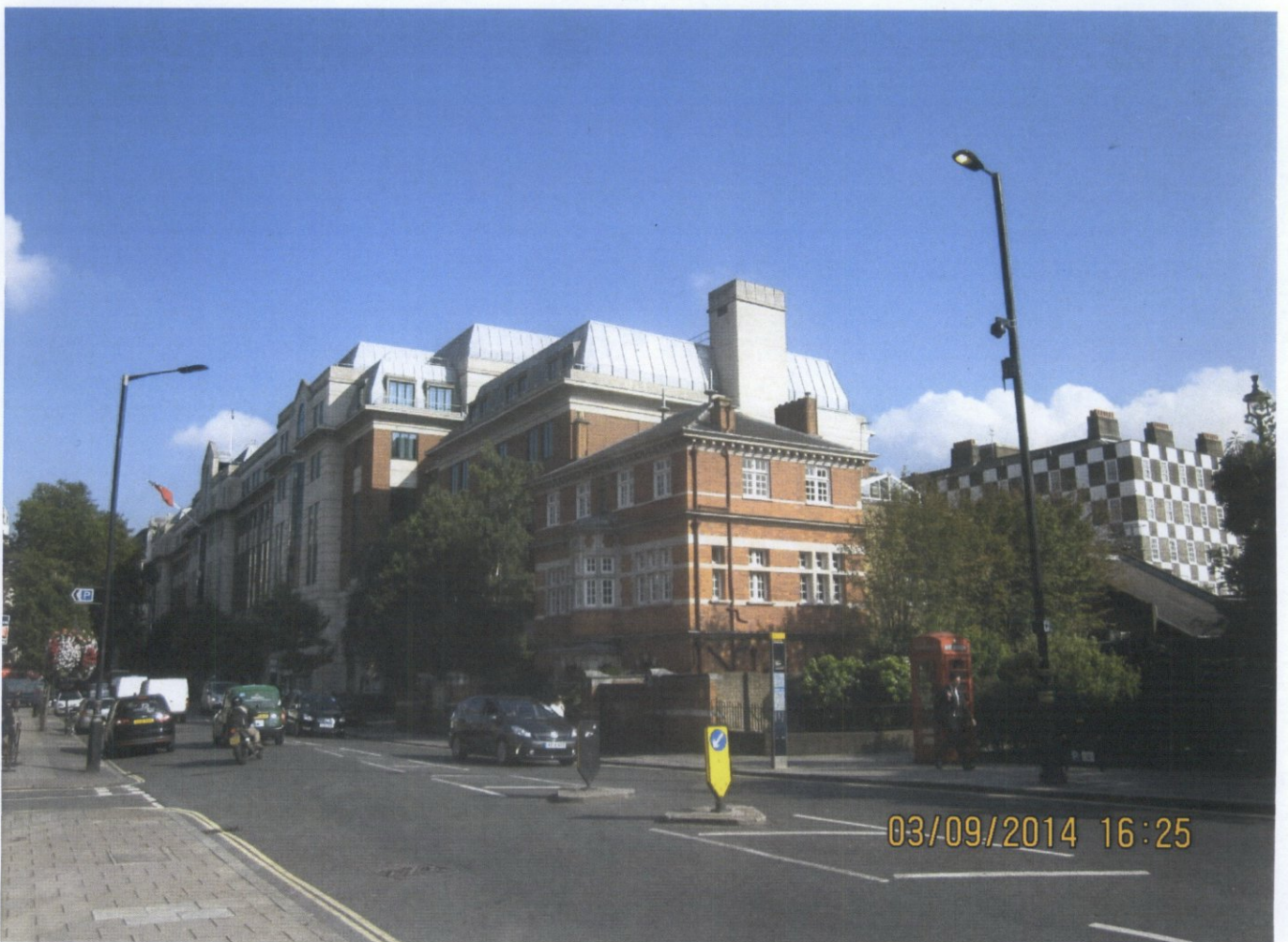
FROM HARBOR ROAD SHOWING WEST ELEVATION OF ABADY HOUSE
