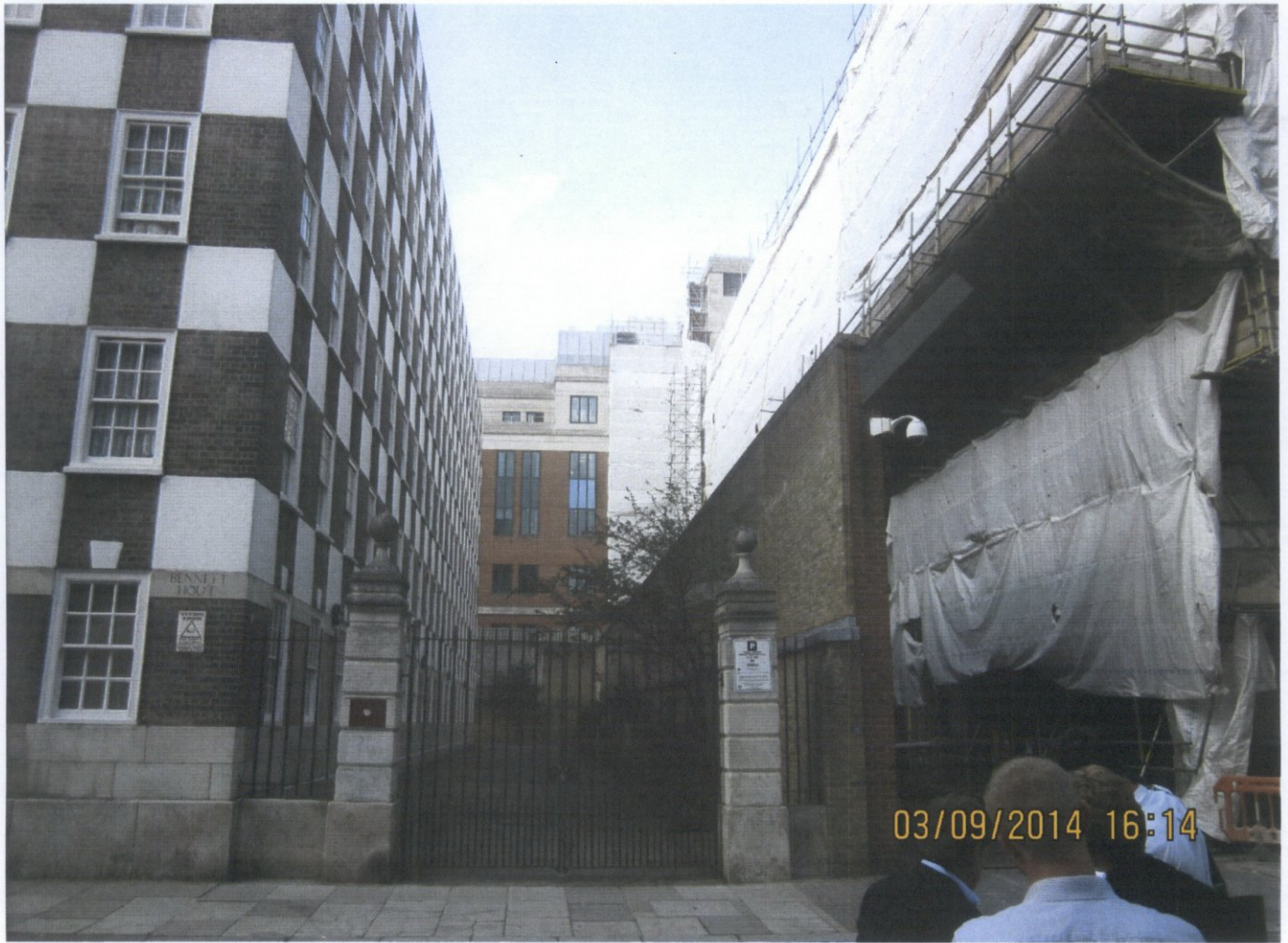
TO NORTH SHOWING ACCESS TO SERVICE ROAD AND BENNETT HOUSE
