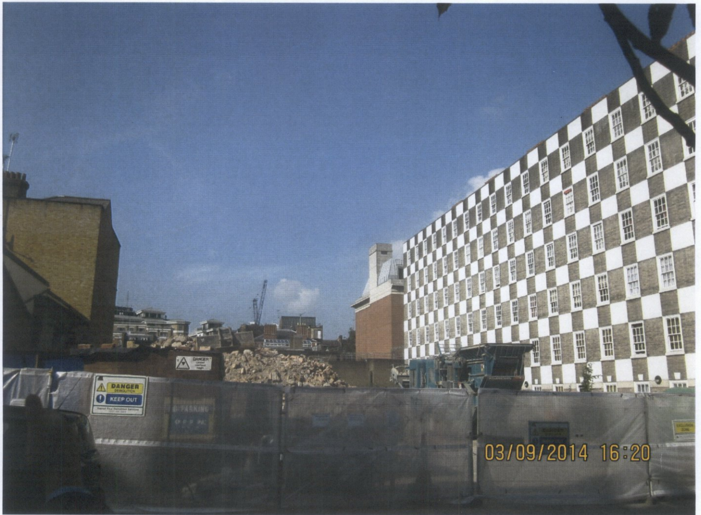
FROM PAGE STREET SHOWING WEST ELEVATION OF ABADY HOUSE
